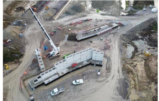
Precast concrete bridge abutments are installed at Station Road
